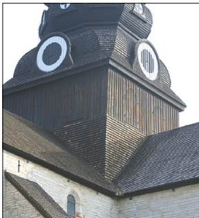
Wood shingles treated with pine tar on the roof of a Swedish church.
